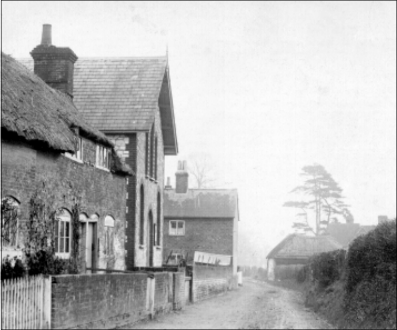
Froyle Methodist Church and Chapel Cottages at the turn of the century
